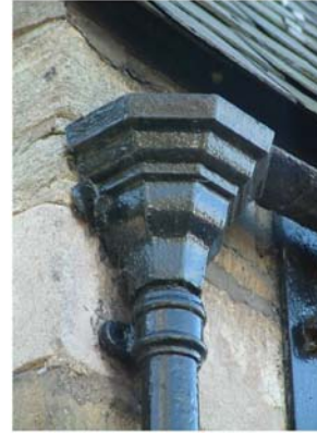
Cast iron rainwater pipe
