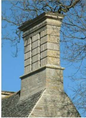
Rusticated chimney stack
